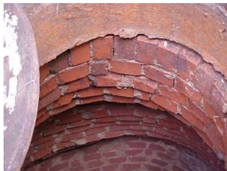
Typical older type manhole
