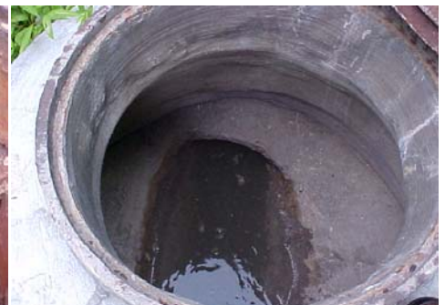
Manhole after rehabilitation.
